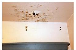
A leaky ceiling in closet that stores computer equipment may not withstand the predicted heavy rain. The closet is between the front lobbies.
